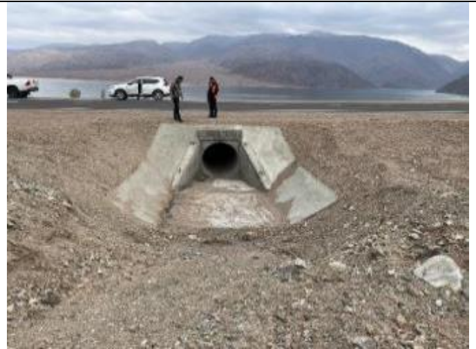
Photo 104. Lot 1: Culvert cleaning, km 33+869.
