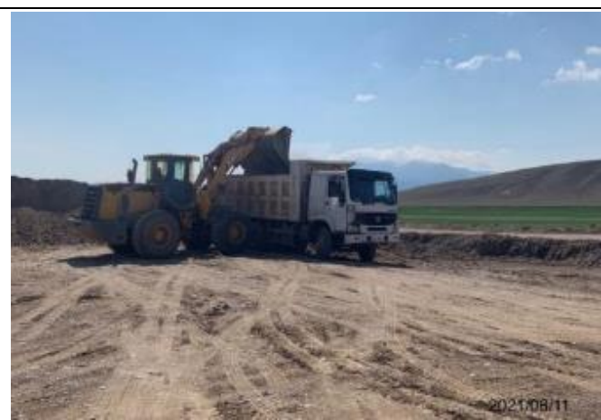
Photo 34. Quarry at km. 81+200, loading of moistened material.
