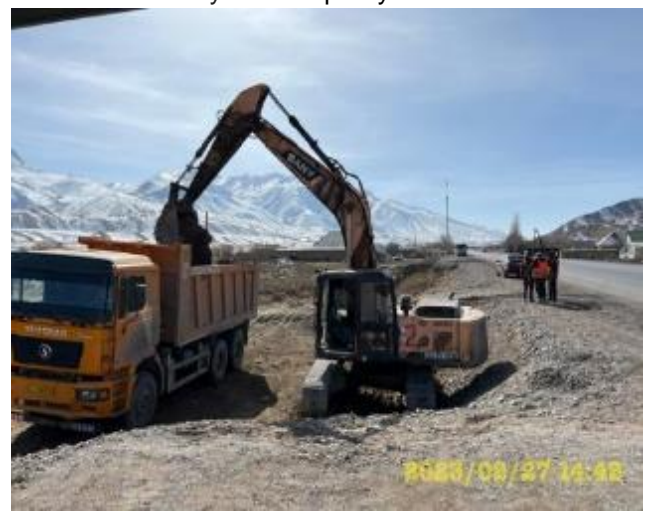
Photo 16. Lot 2. Removal of soil and vegetation layer from sidewalk area
