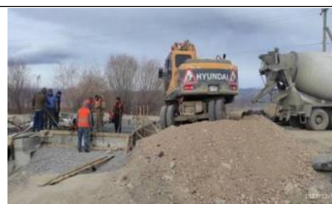
Photo 89. Concrete pouring of transition slab 1 km 68+044.
