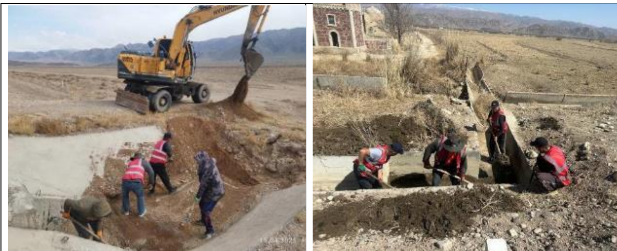
Photos 5, 6. Cleaning of culvert channels and concrete chutes.
