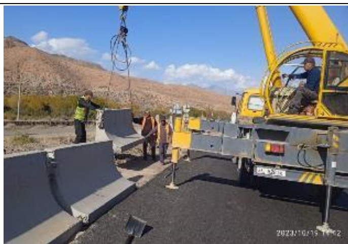
Photo 110. Installation of parapets at km.11+200.
