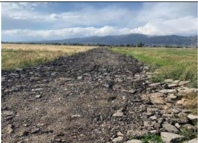
Photo 58, 59. Improvement of peripheral street with old asphalt (laying and leveling) in Cholpon village.
