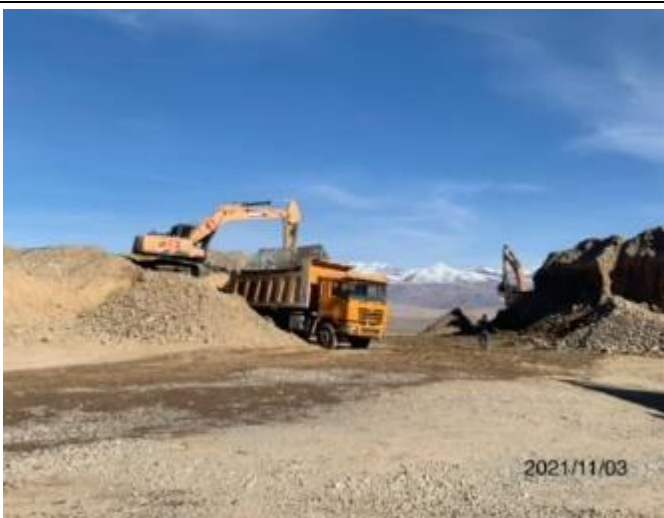
Photo 33. Quarry at km.75+400. The material is being mined, after it has been moistened.
