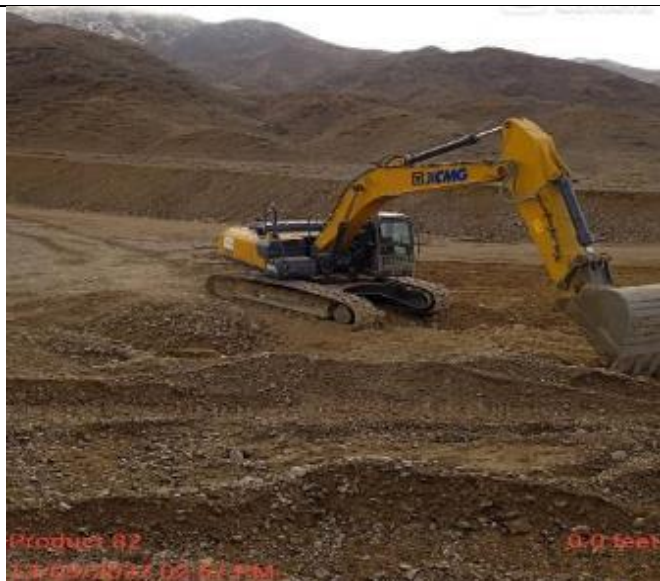
Photo 29. Quarry technical leveling at km 34+240 and bringing quarry slopes to a safe condition.
