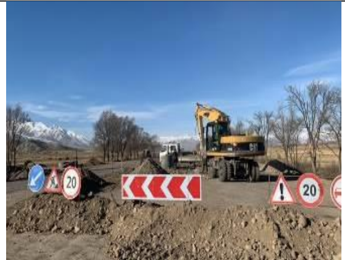
Photo 98. Lot 1. Compaction of soil backfill of culvert at km 20+670.
