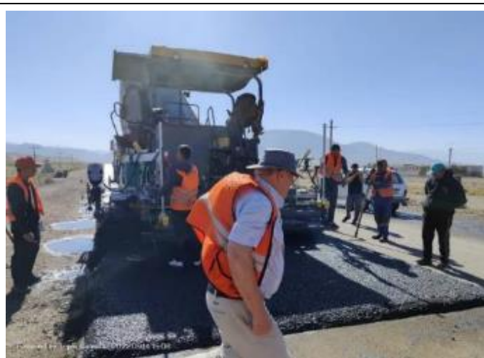
Photo 75. Lot 2. SMA arrangement km 81+675-82+000 RHS.
