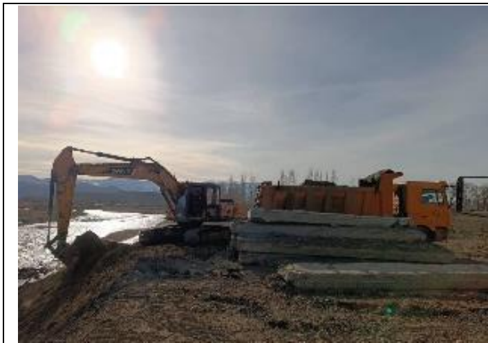
Photo 90. Dismantling of temporary bridge for bypass road at km 62+500 over Joon-Aryk River.
