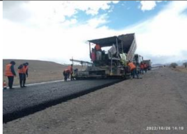
Photo 75. Lot 2. SMA arrangement km 81+675-82+000 RHS.
