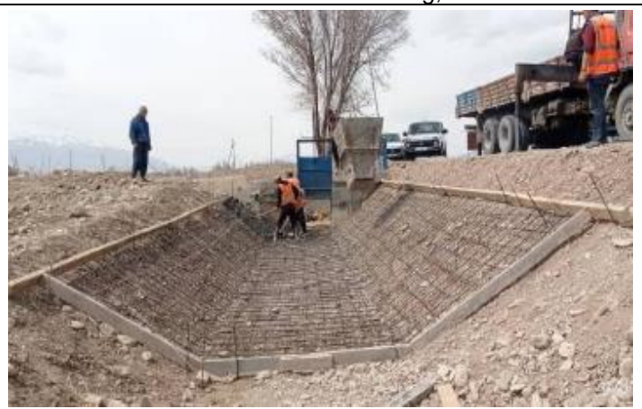
Photo 106. Lot 2. Pouring of concrete for slope reinforcement at km 64+860.
