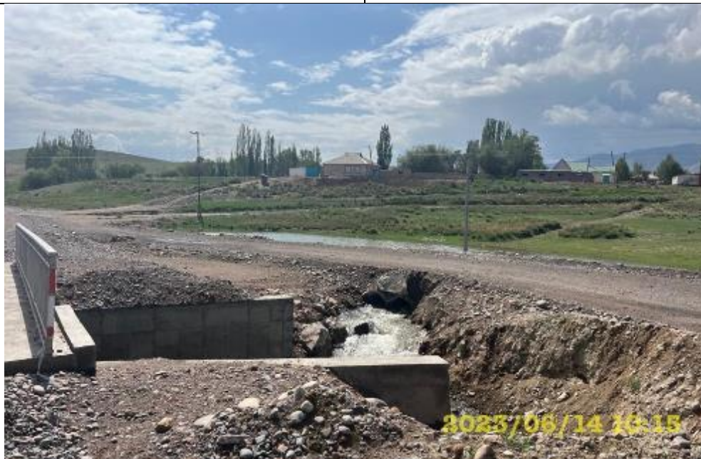
Photo 94. Lot 2. Mukandyn-Suus River bridge, km. 68+040. There are no protective measures to prevent soil from entering the river during construction works.
