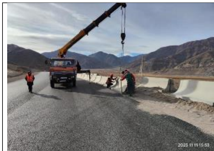
Photo 109. Installation of parapets on 40+700-40+870 RHS.
