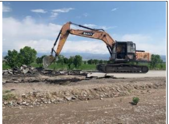
Photo 50. Scarifying of asphalt concrete pavement at km 74+550.
