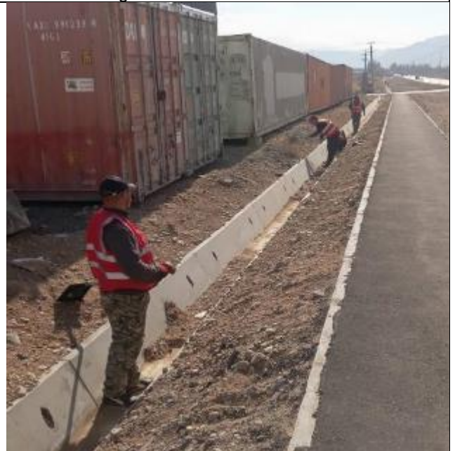
Photos 3, 4. Cleaning of sidewalks and drainage chutes.
